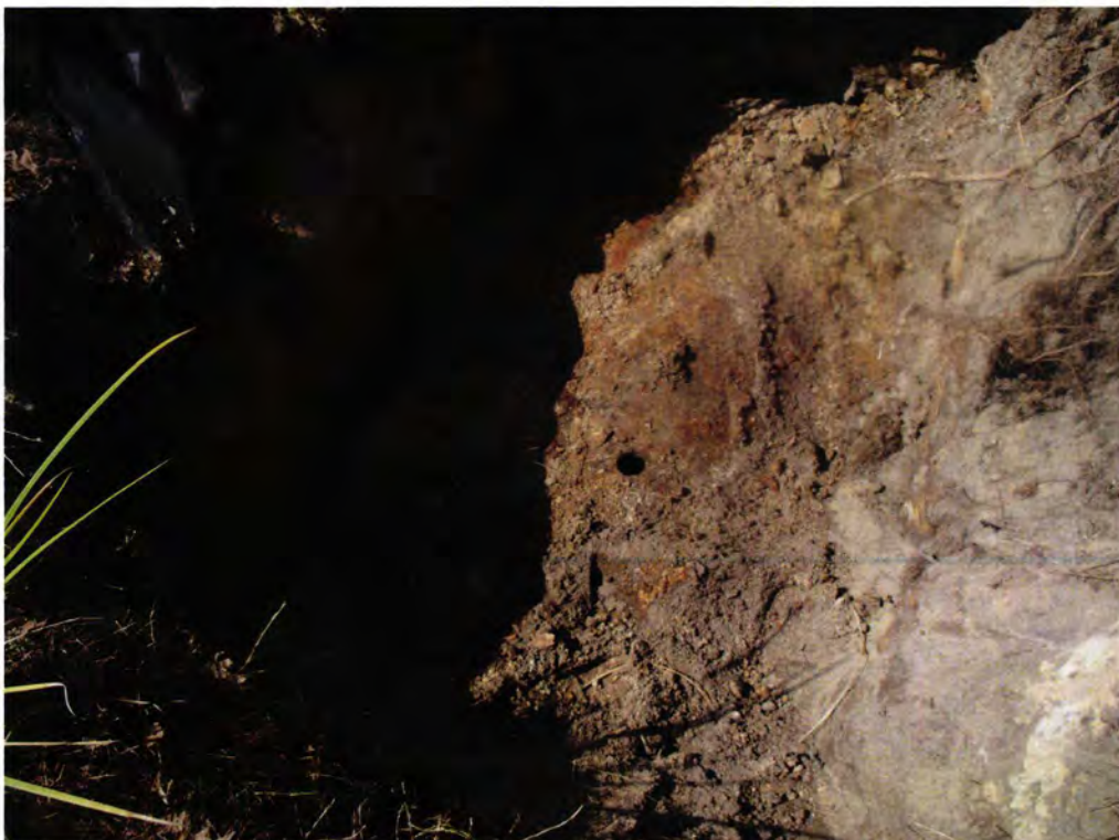
Picture 2: UST 306Ash removal in progress.
